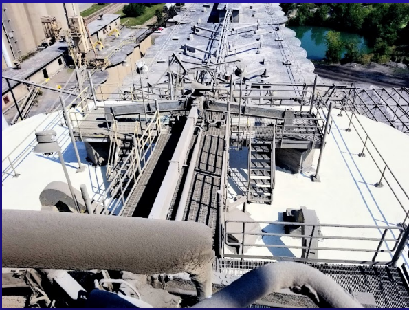
Poly-Armor Over Concrete Silo
