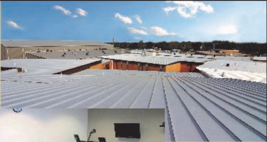
Cole Camp R-I School Re-roof
