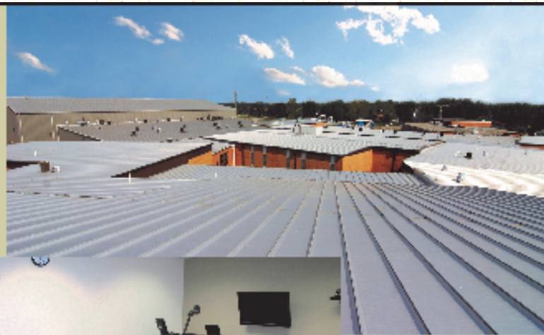
Cole Camp R-I School Re-roof
